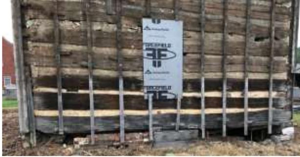
Detail of size of logs, notching and 19<sup>th</sup> century chinking, east elevation
