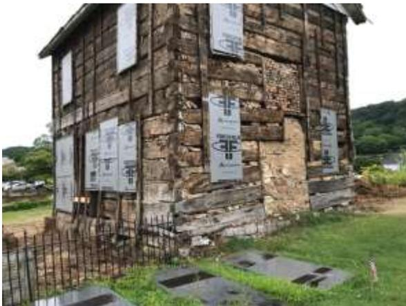
This image shows the historic west and north elevations. Note the interior chimney, a very unique feature of the building. Also note where it is located on a slight grade, a typical feature of Pennsylvania log construction of the late 18<sup>th</sup> century.
